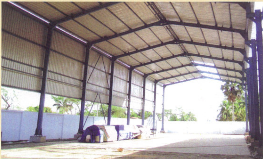
PEB Structure with RHS Purlines.
